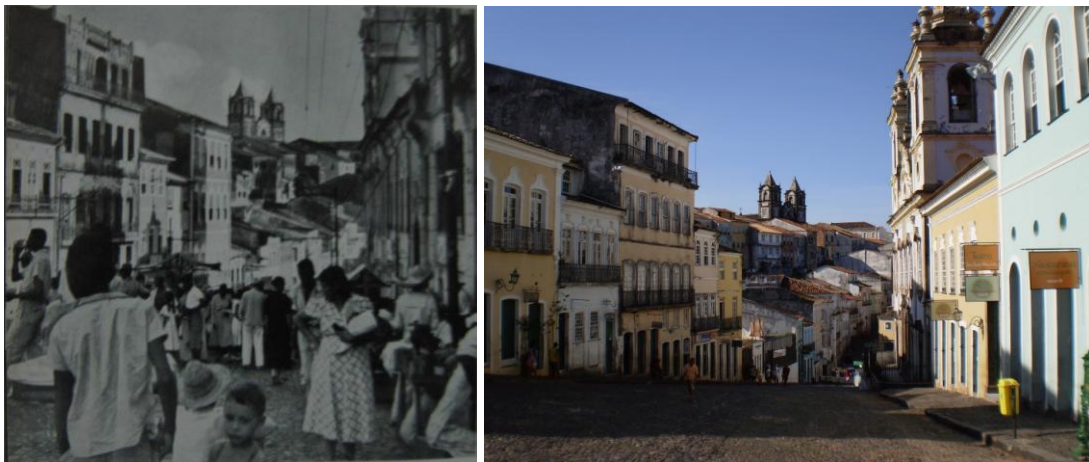
Figures 13 & 14: The busy streets of Largo do Pelourinho in the 1950s (left), Photograph by Alice Brill. The empty façades of the Largo do Pelourinho in 2009 (right), Photography by Puneet Singh.
